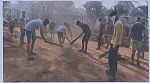
Cleaning of roads
