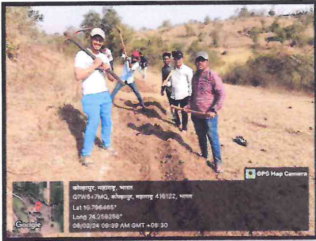
Conservation of water resources - Continuous Contour Trench (C. C. T.) Method.
